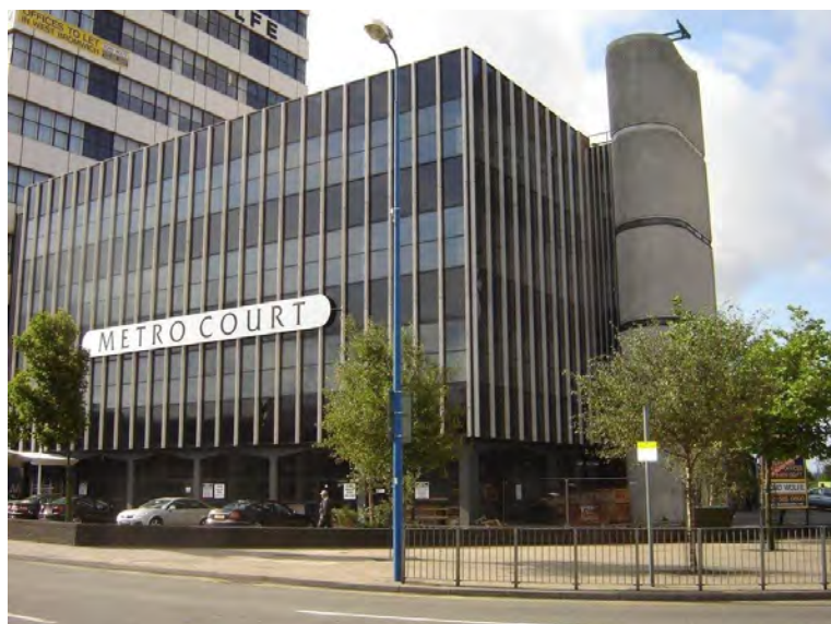
METRO COURT, WEST BROMWICH
